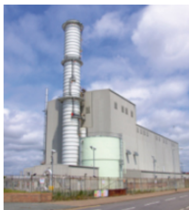
Great Yarmouth Power Station
